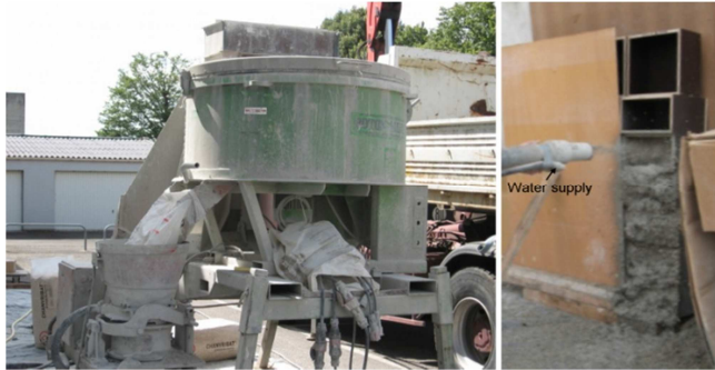
Figure 1. Spraying method (left : mixer, right : spraying hose)
