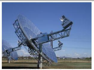
Figure 1- Dish-Stirling engine Power plants
