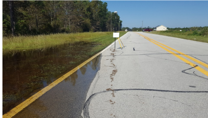
Figure 16: Street view of the debris line high water mark in Figure 14.
