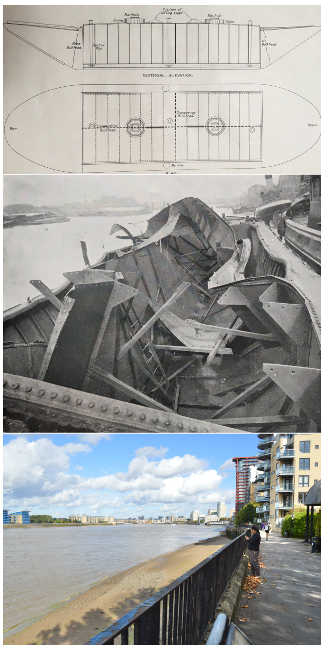
FIG. 1. The explosion of the petroleum barge, Warwick , on 24th September 1920. Above: the design of the barge, showing its petrol tank. Centre: the remains of the Warwick after the explosion. Both images reproduced from the accident report 16 . Below: the same view a century later, on 24th September 2020; the Thames is now a post-industrial river.
