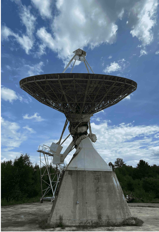
Figure 2. ARO 10-m telescope; photograph taken in September 2020. The backplane and CHIME feed are visible at the telescope’s focus. The feed in the paraboloid focus is slightly offset towards the vertex.
