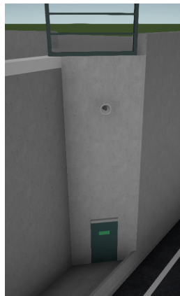
Figure 6.21: Closed head door leading to the central corridor at the tunnel entrance.
