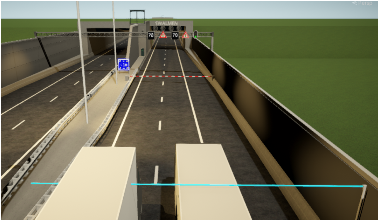
Figure 6.16: Height detection system with a truck that is too high (left) and a truck that is allowed to enter the tunnel (right).
