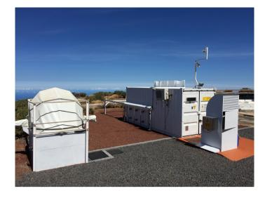
**Figure 2.** WLGSU configuration at Observatorio del Roque de los Muchachos next to the William Herschel Telescope, with the receiver (Rx) dome (left) and the sliding-roof container accommodating the laser beam transmitter (Tx).
