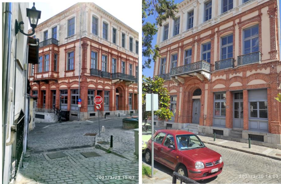
Figure 2. Outside view of M. Hatzidakis' residence.
