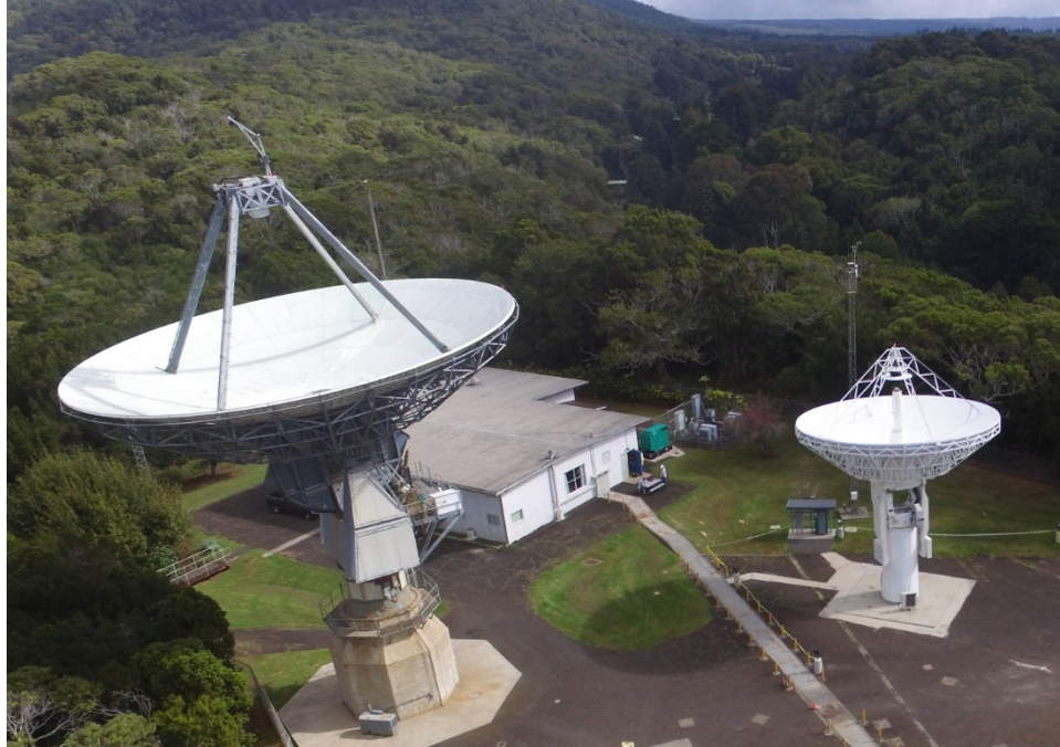
Fig. 1 View of the Kokee Park Geophysical Observatory (KPGO) showing the 20 m legacy antenna (left) and 12 m VGOS antenna (right); source Chris Coughlin and Kiah Imai, KPGO
